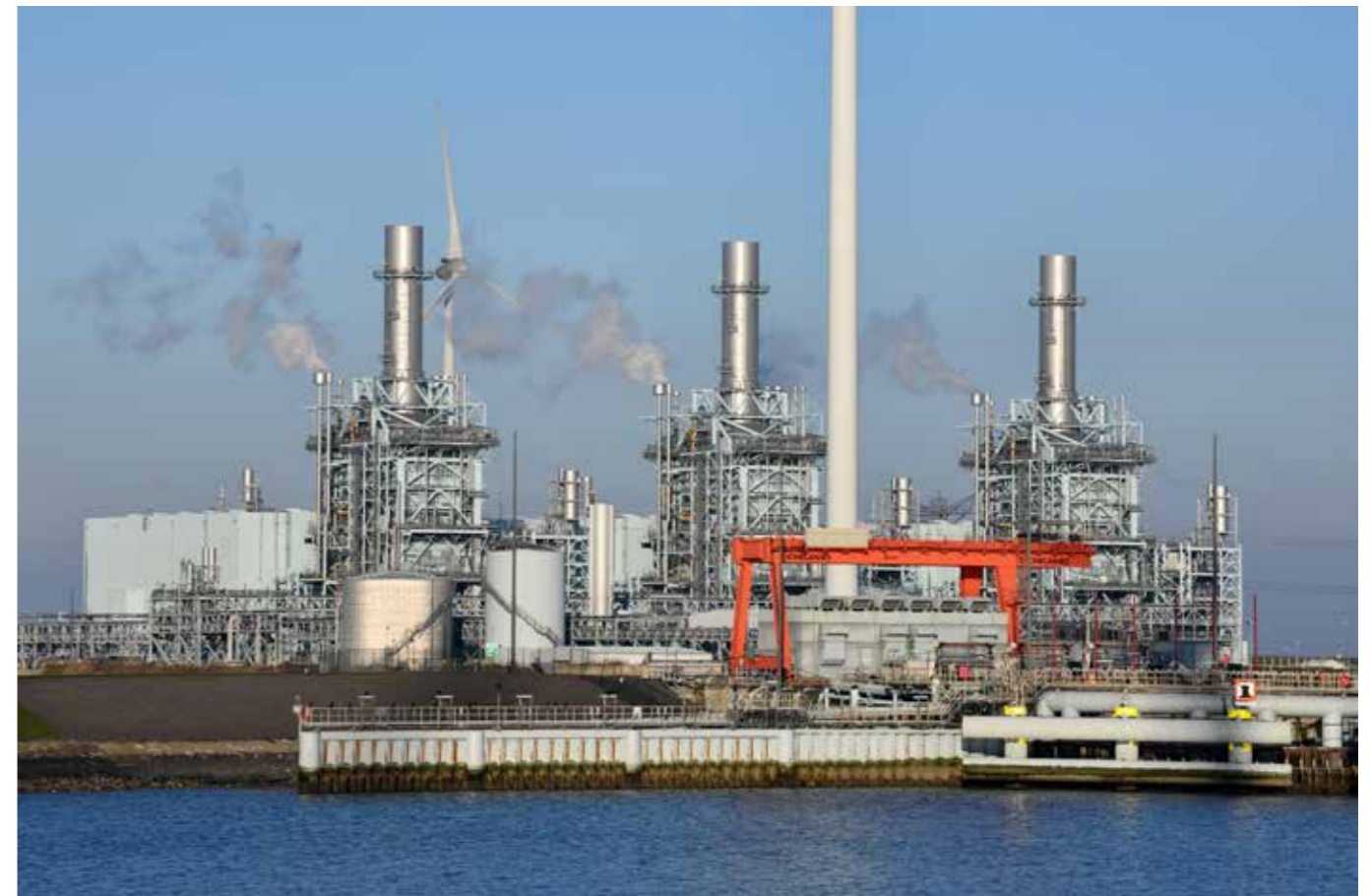
RWE EEMSHAVEN MAGNUM
